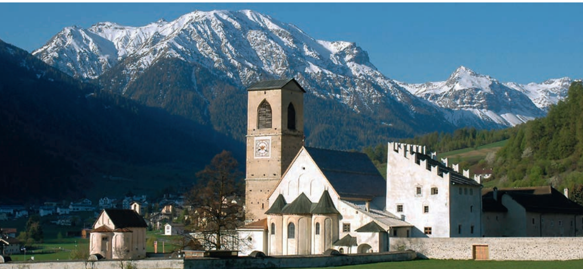
Benedictine convent of St John at Müstair with the Chapel of the Cross, Convent church and Planta tower | Convento Benedettino di San Giovanni a Müstair con la Cappella della Santa Croce, Chiesa del convento e Torre Planta © Stiftung Pro Kloster St. Johann in Müstair
